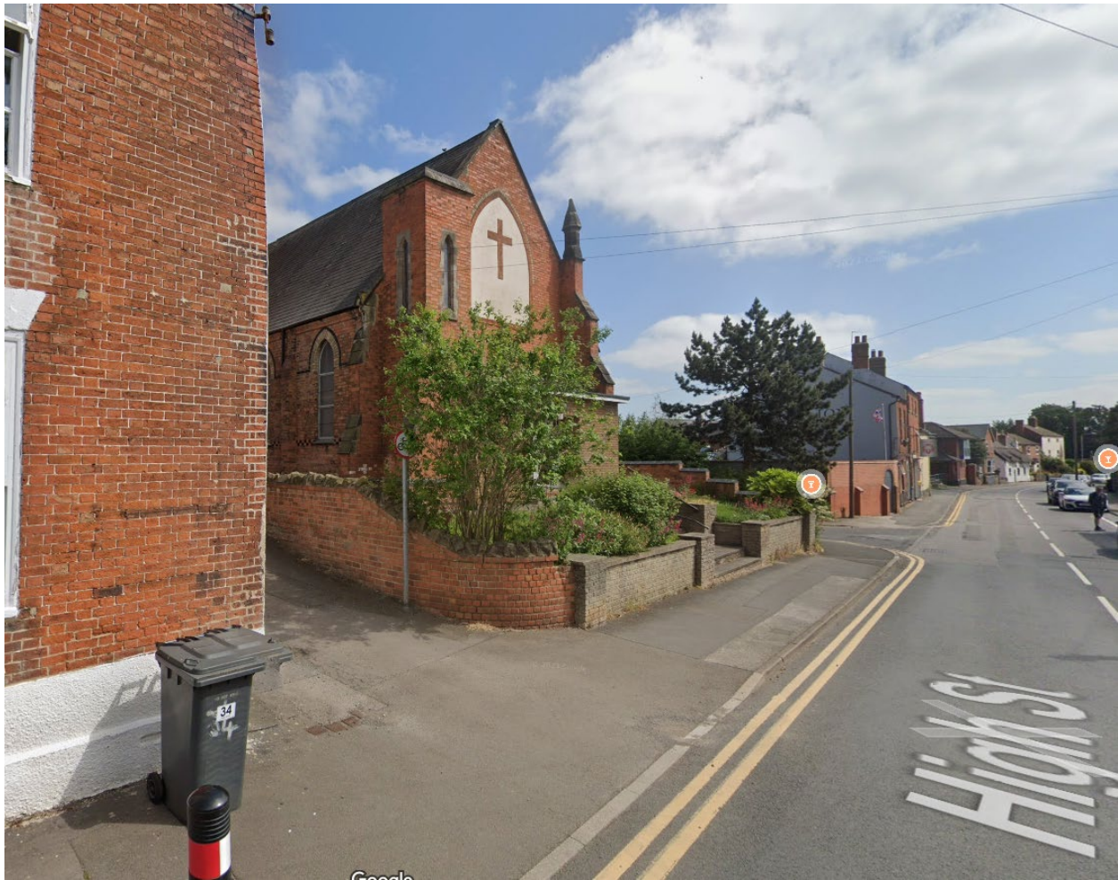
View looking east on the High Street standing outside no. 34
